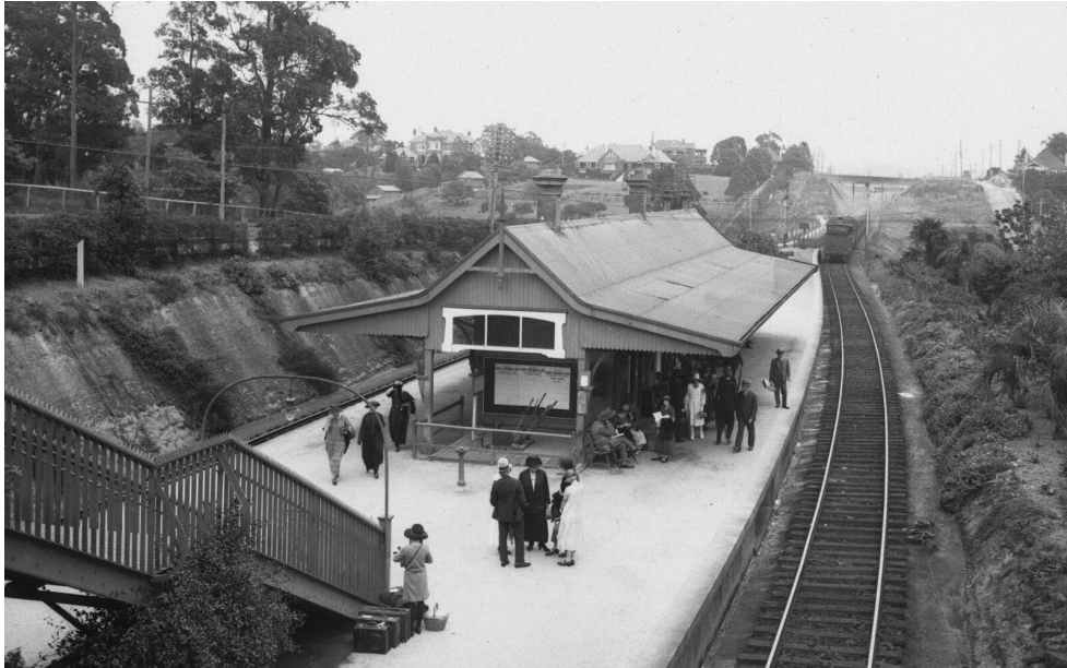
Above: Killara Station and surrounding housing in 1924 (Source: State Archives, https://search.records.nsw.gov.au/permalink/f/1ebnd1/ADLIB_RNSW115668623 )
