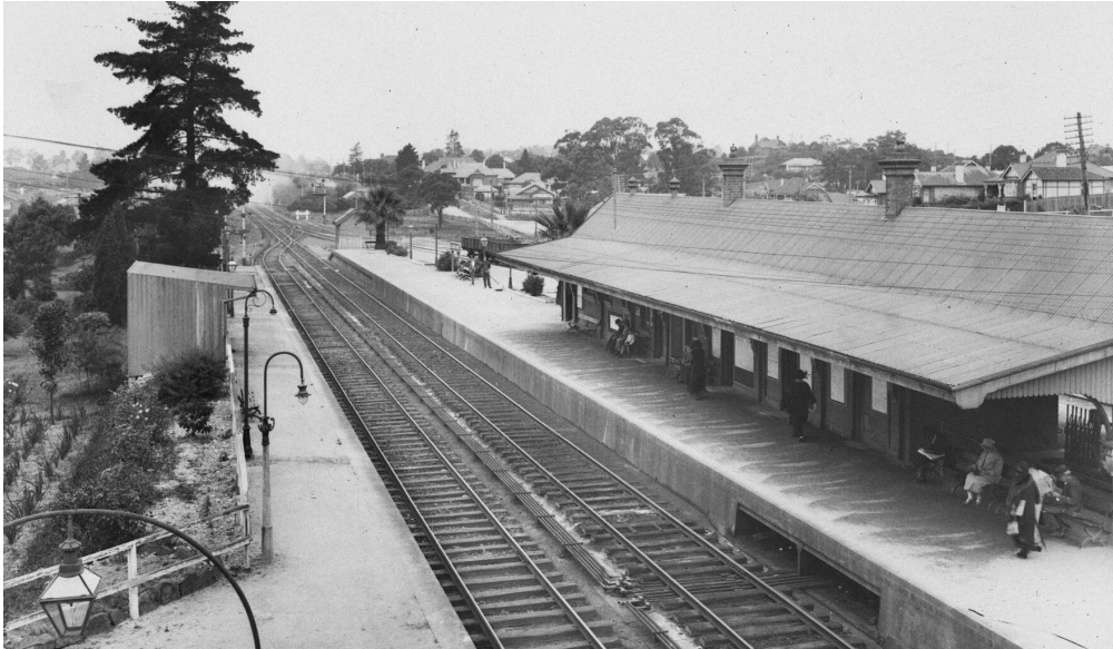
Above: Gordon Station and surrounding housing in 1924 (Source: State Archives, https://search.records.nsw.gov.au/permalink/f/1ebnd1/ADLIB_RNSW115668621 )
