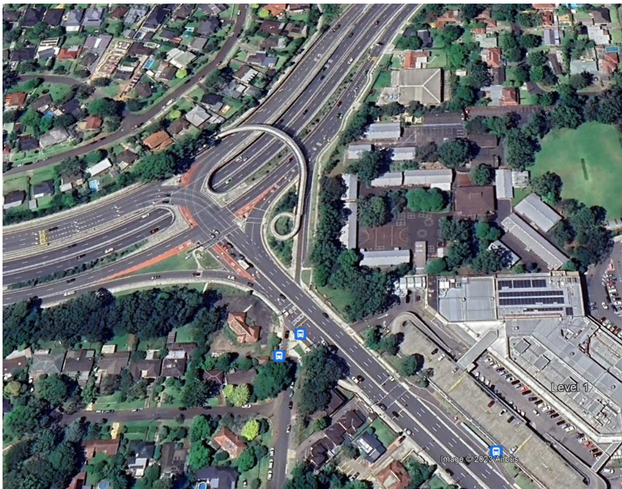
Figure 3.10 – Photo showing new intersection with Warringah Road and Forest Way
